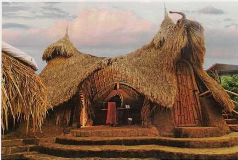
Teacher accommodations are also built almost entirely from bamboo (top & far right). The unusual roof and building shape is a bathroom (above).
