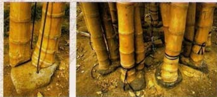
This sweeping arch is the covered way of a bridge that crosses the river running through the centre of the school (far right). A classroom of another kind — one that can be air-conditioned if needed — is used by young children (top photo, this page). The foundations of buildings display unique construction techniques: a concrete slab is buried with only an iron rod left protruding. That passed through a stone and into the bamboo pillar in a manner that leaves both concrete and iron unseen in the finished product (above).
