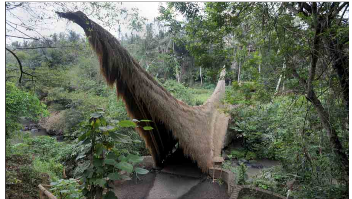
The sculptural all-bamboo bridge that crosses the Ayung River linking the two sides of The Green School campus.
